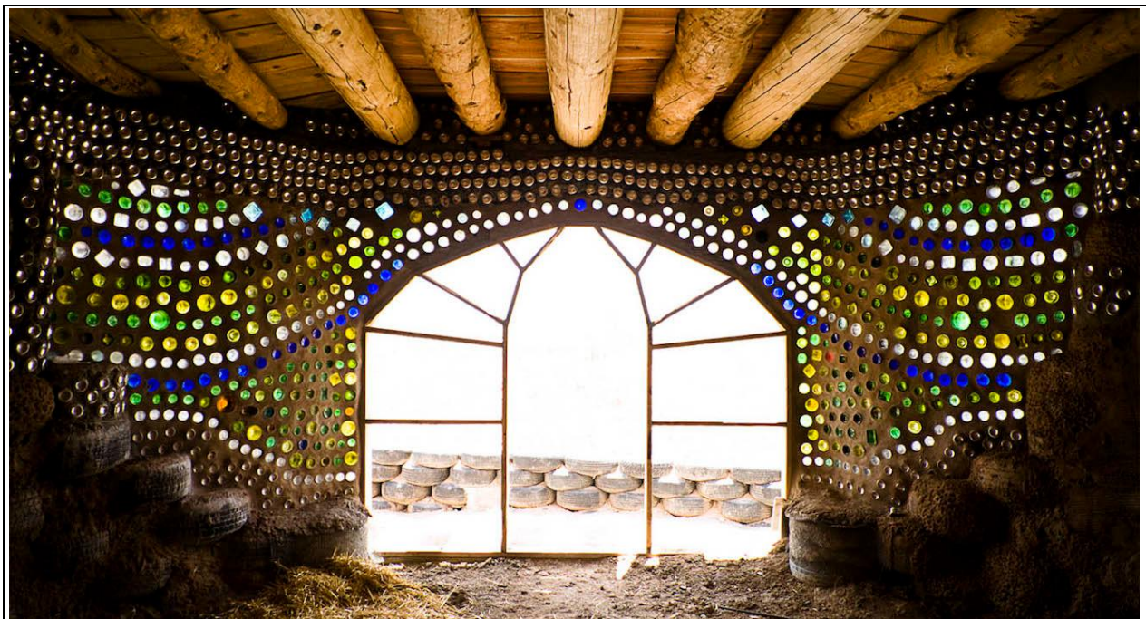
Figure 15: Picture of an Earthship glass wall, classic in this type of building
